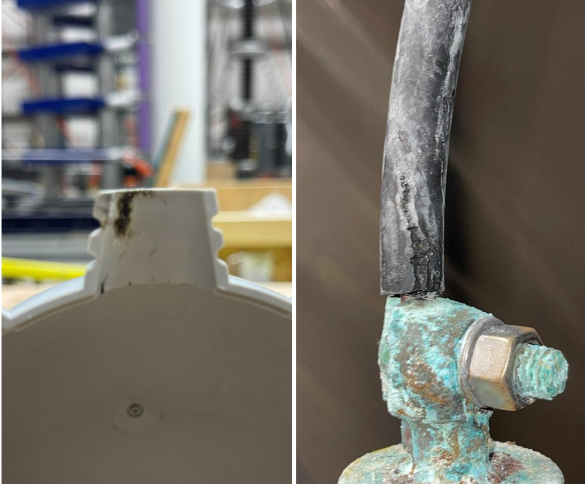
Figure 8 – Detail of stain in Sample B-2 (left), where no tracking or measurable erosion were present, and cable that eroded (right) causing the black stain on the sample.
